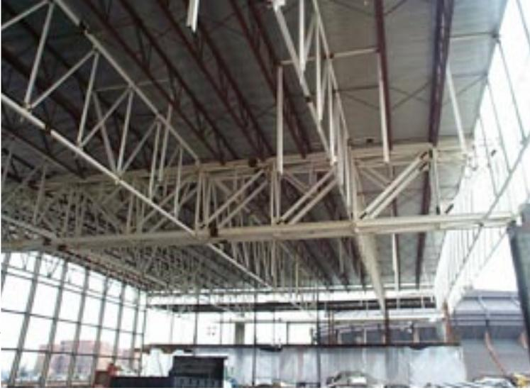
Twin steel girder trusses, consisting of wide-flange chords and double angle webs, span between the mast columns to support long-span joists on each side of the exhibit hall roof.
