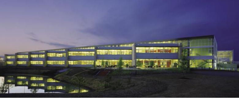
The steel-framed "saw tooth" design of the exterior walls was created to reorient the building, which had faced southwest, to essentially face south. This allows more daylight into the office spaces while providing relief from direct afternoon sun.
