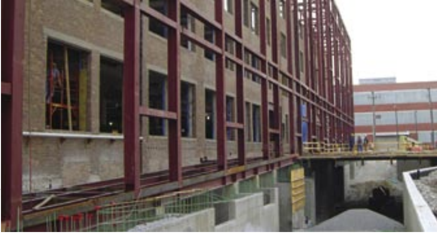
Steel framing for the atrium façade is visually appealing and provides the needed stiffness to limit deflection under design wind loads.
