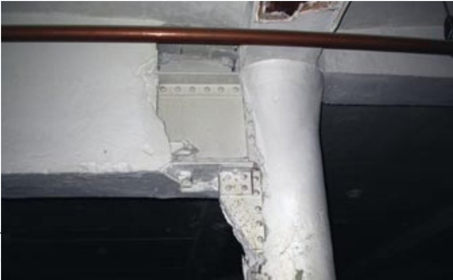
The original steel members are typically built-up sections consisting of flange angles riveted to web plates.
