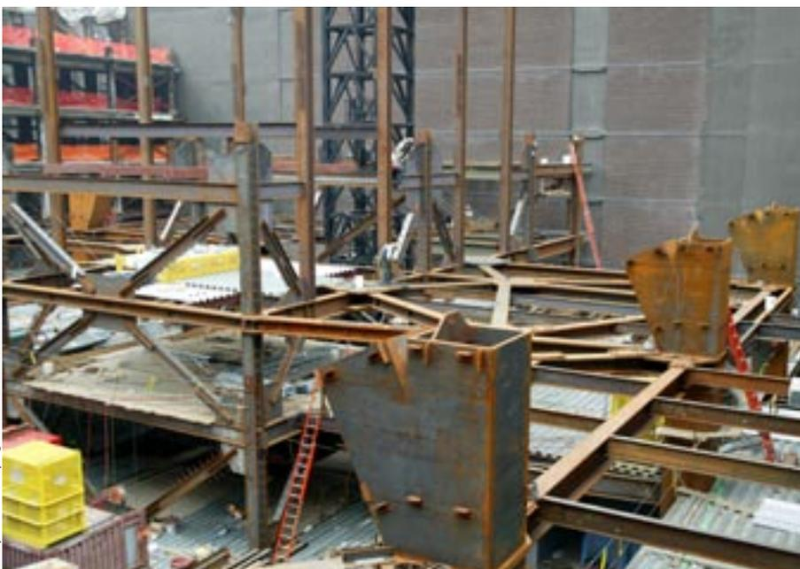
with one or two points in trying to make all the bolts fit because there were so many bolts coming into some of the corner nodes [also called the “bird’s mouth” nodes], but all in all it fit very well. The New York City Erectors Local No. 40 sent a letter saying it was some of the best fabricated steel they’d ever seen for this complex a structure.
