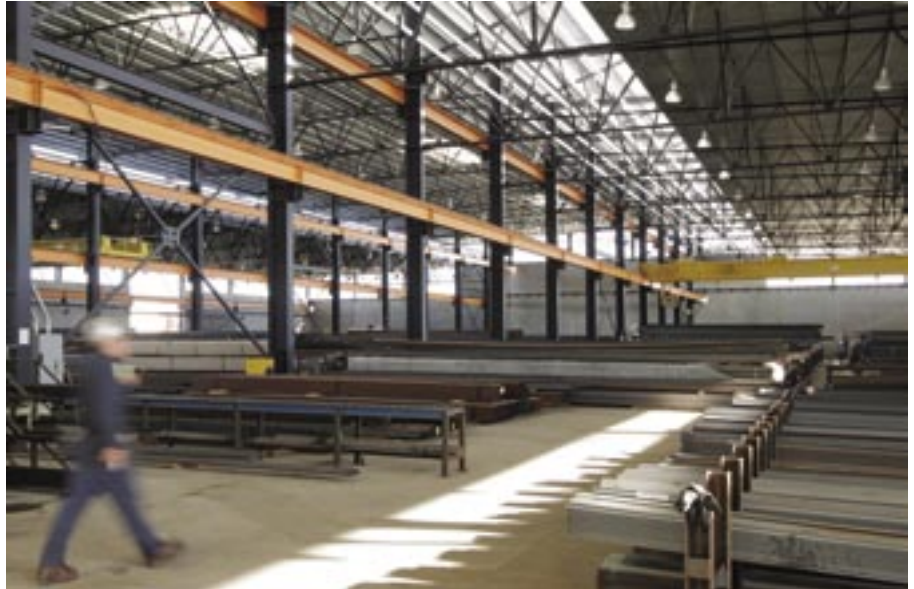
The interior of the Triple-S Steel Supply facility in San Antonio, Texas.
