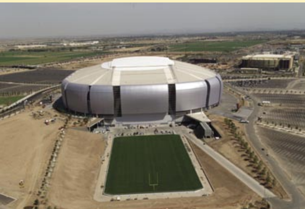
Operable field under construction in outboard position.
