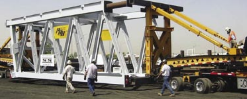
Brunel truss box sections in transport.
