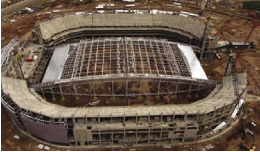
Superlift assembly prior to lift.
