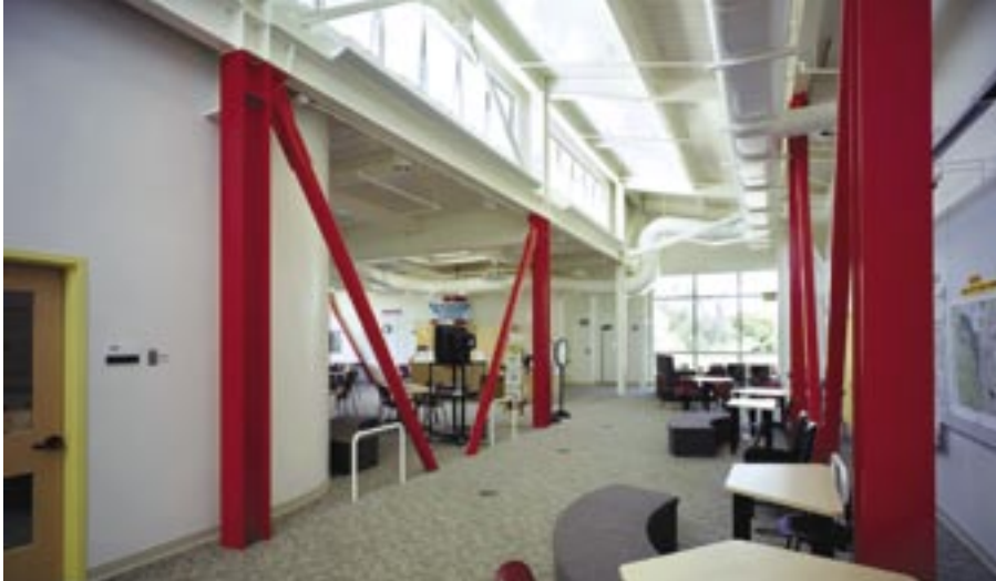
The braces are prominently featured as interior architectural elements.
