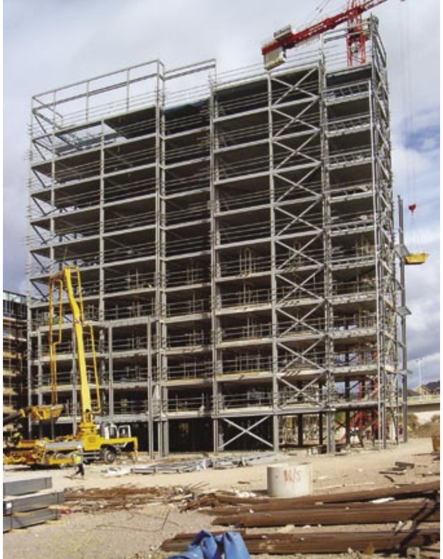
Steel frame erection completed a week ahead of schedule.
