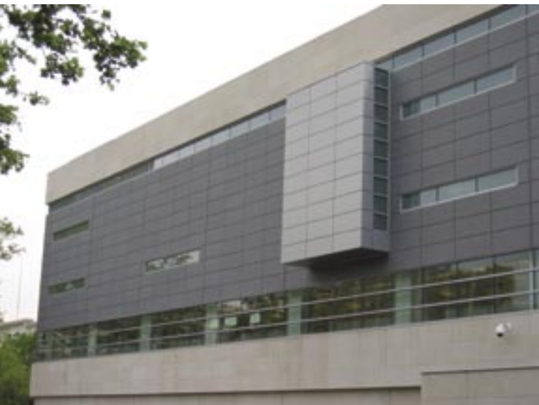
The completed limestone exterior is shown in this view of north facade.
