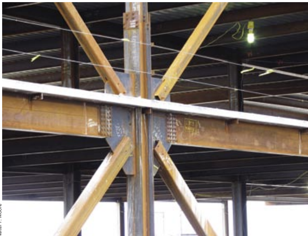
Because the brace connection forces were typically significantly larger than the beam force, the floor beams connect to continuous gusset plates, instead of interrupting the gussets.
