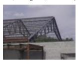
spans up to 130 ft, are our feature products. Our joists are formed of small cold formed channels to provide individual web members for most steel joists spanning over 30 feet.
