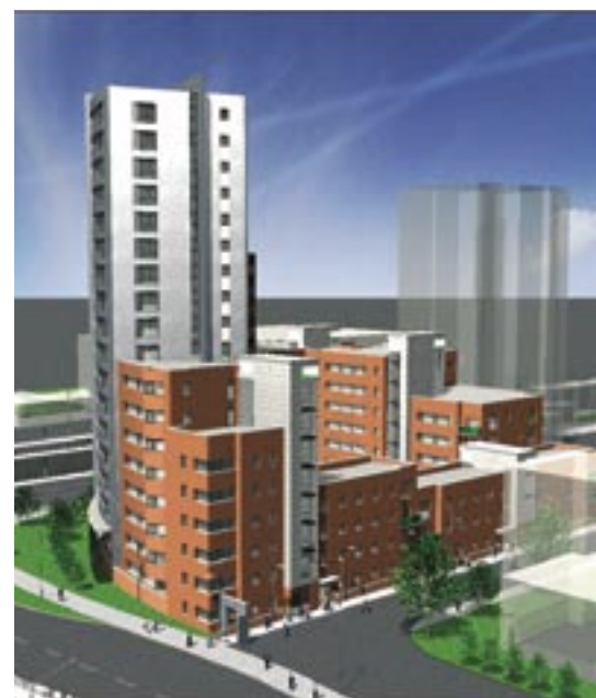
The Birmingham 1 project features an 18-story residential tower with a steel core.
