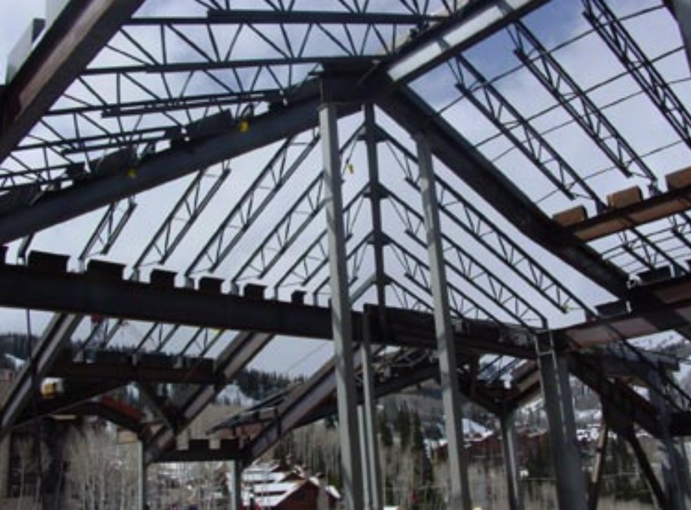
The multi-gabled roof of the Silver Strike Lodge is framed with open web steel joists and wide-flange beams.
