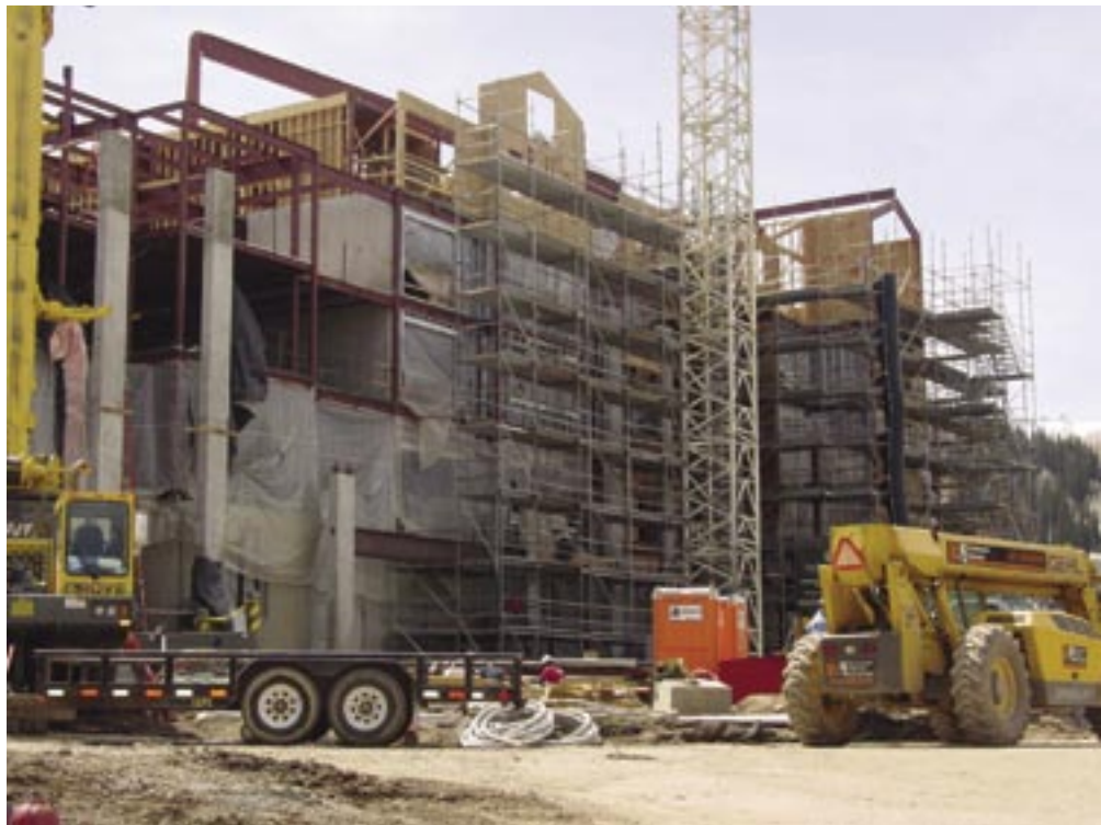
The Grand Lodge (shown) differs from the Silver Strike Lodge in that its gabled roof is framed in wood.
