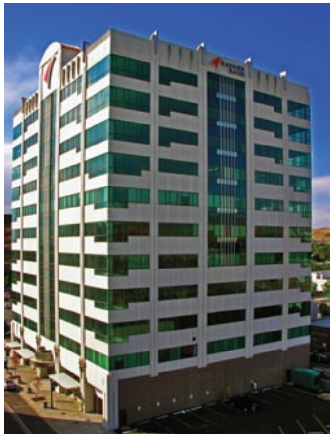
The 11-story Banner Bank Building features 45-ft clear spans for office layout flexibility.
