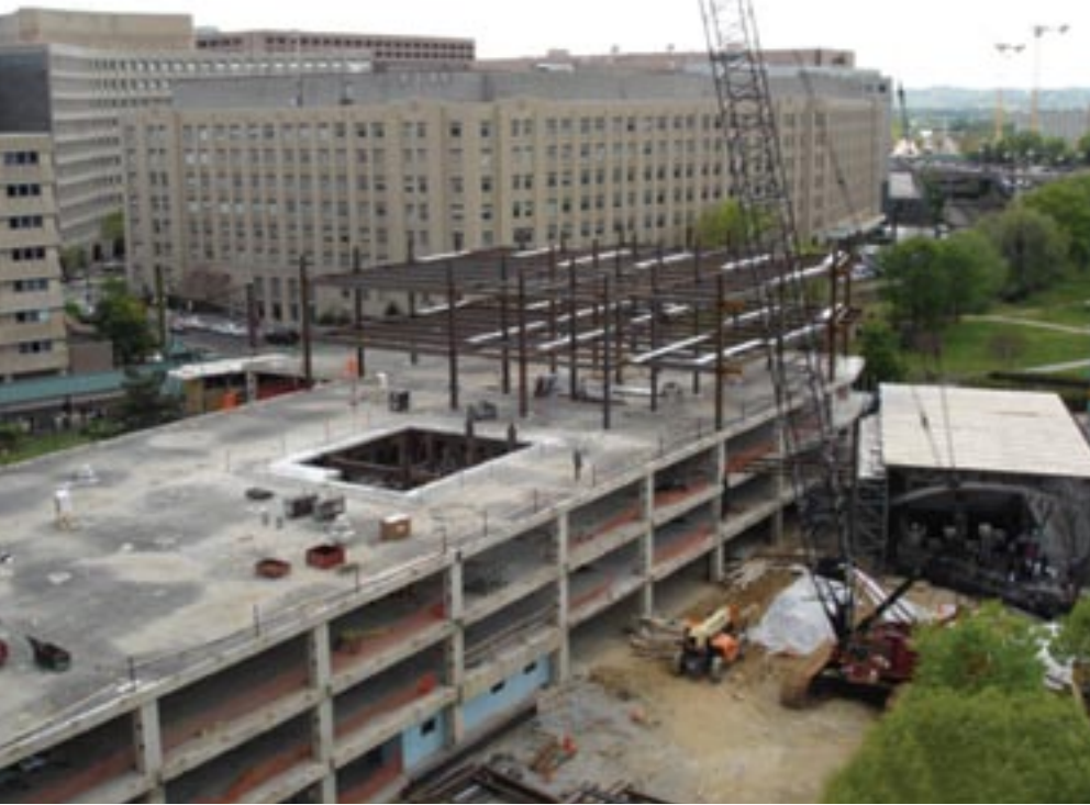
Seven floors of steel-framed offices were added atop this three-story concrete structure from the 1970s.
