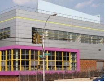
To lighten loads on the existing perimeter footings, which support the new second floor, the original masonry exterior was removed and replaced with a metal panel and glass curtain wall system.
