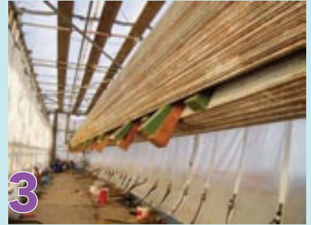
Wedges are driven into the center of the cable so that they can be inspected.
