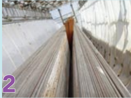
Wedges are driven into the center of the cable so that they can be inspected.
