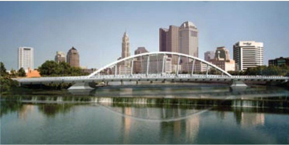
The new Main Street Bridge in Columbus will be completed in 2009.
