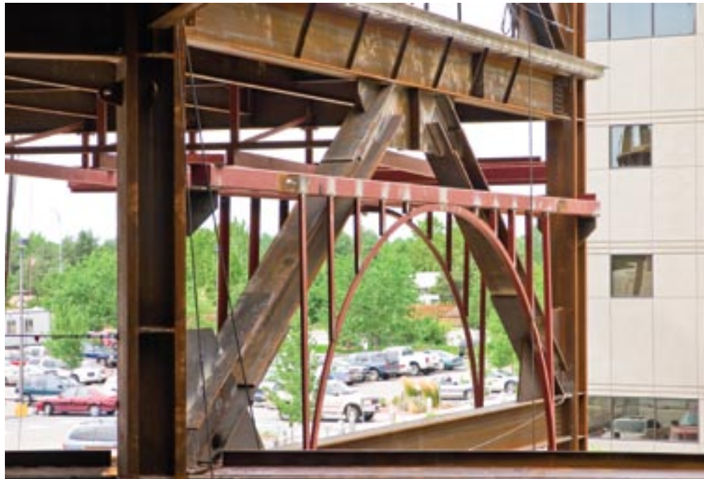
The lateral system is formed by a combination of braced frames (shown) and moment frames.
