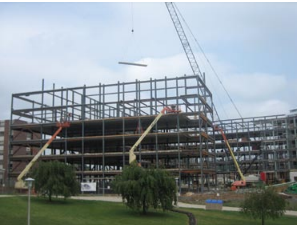
Steel erection at Kutztown University occurred this summer. Lateral bracing is provided by chevron braces strategically located to avoid window locations.
