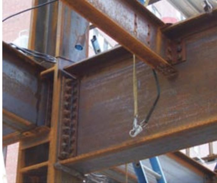
Preheating top flange of moment girder before welding in cold weather conditions at Maine Medical Center.
