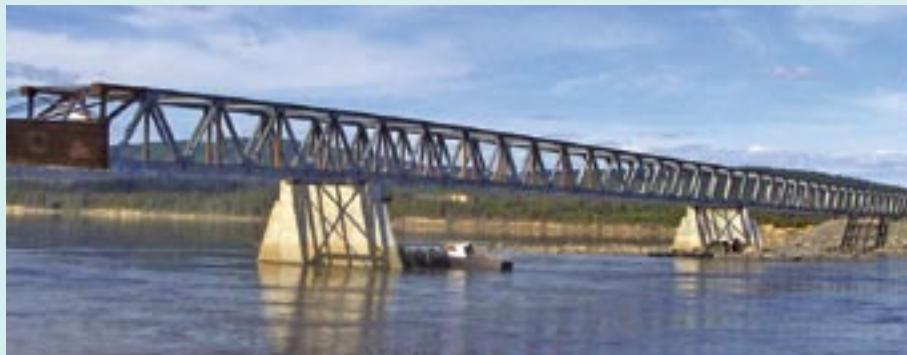
ery and erection schedule. This includes the deck steel, railings, and structural steel. The bridge is comprised of three spans in excess of 400 ft each, as well as about one-half mile of approach causeways.
