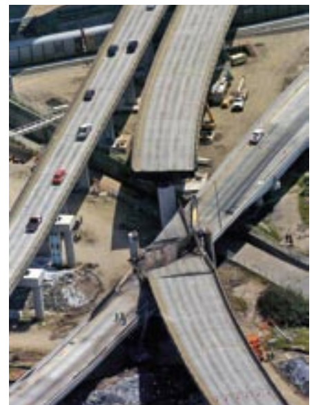
The steel box beam bent cap spanning the I-880 connector collapsed in the estimated 1,500 °F fire.
