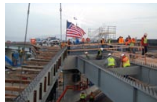
Built-up sections were fabricated with thicker web plates to minimize the number of stiffeners required. Flange plates were kept constant to simplify fabrication. The bridge reopened to traffic in only 25 days.
