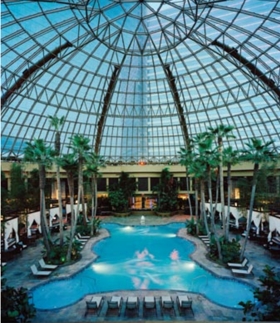
Atlantic City Harrah's Resort and Casino's pool complex (left) features a 208-ft-diameter, 50-ft-tall glazed dome framed with structural steel.
