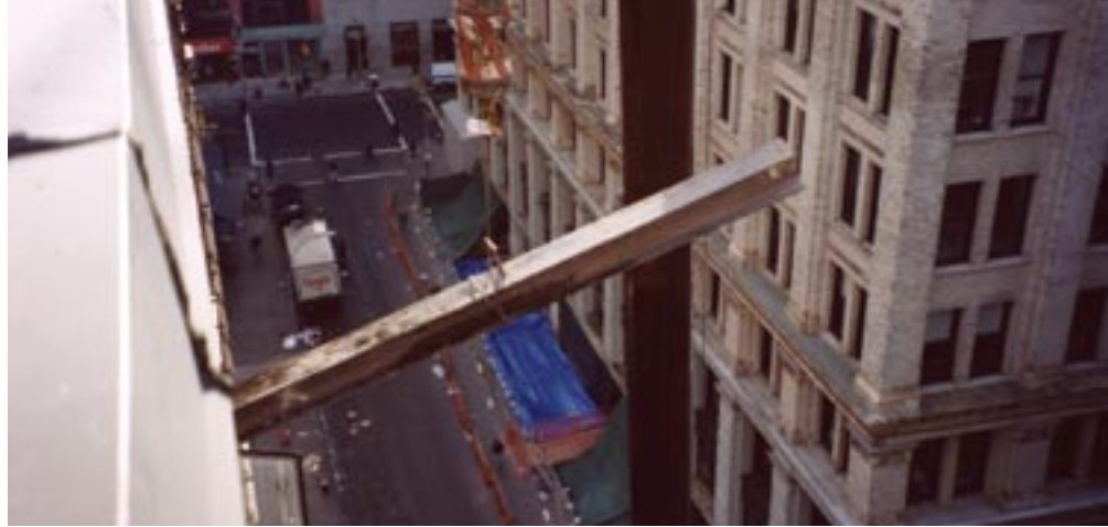
New steel members were lifted by a crane at street level and needled through a 12th-floor window for installation under the main roof.
