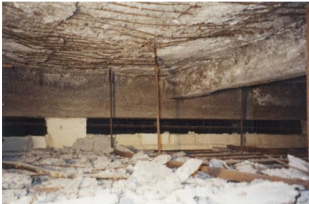
Chunks of the deteriorated cinder concrete roof slab landed on the flimsy stucco ceiling. The ceiling was hung from the same deteriorated roof slab.
