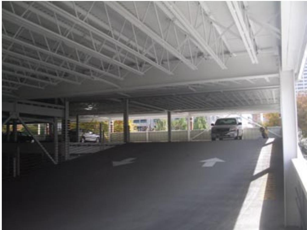
Throughout the garage, new joists were added in between the original joists to decrease the slab's span.
