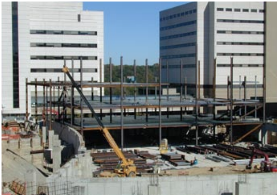
Photos: Douglas Steel Fabricating Corp.
