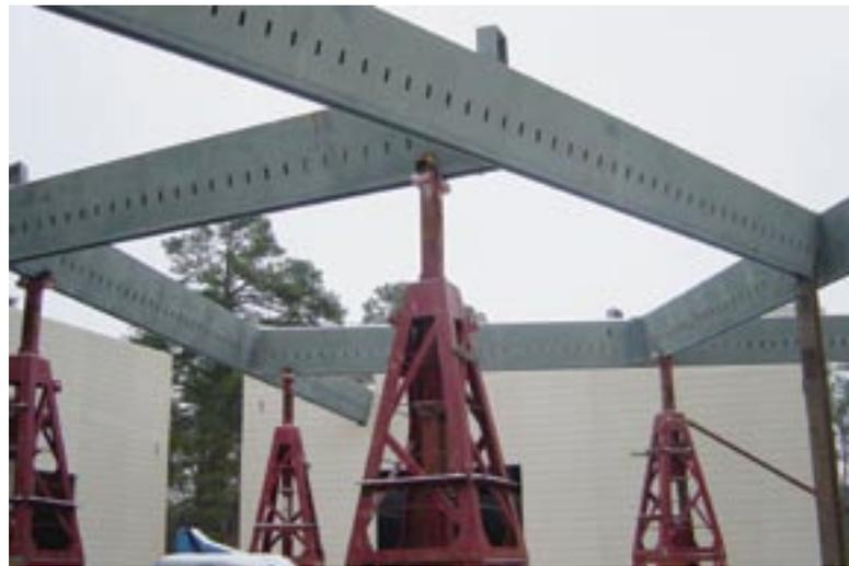
three places—once by the load-bearing concrete walls of the pavilions, and twice by the other beams.
