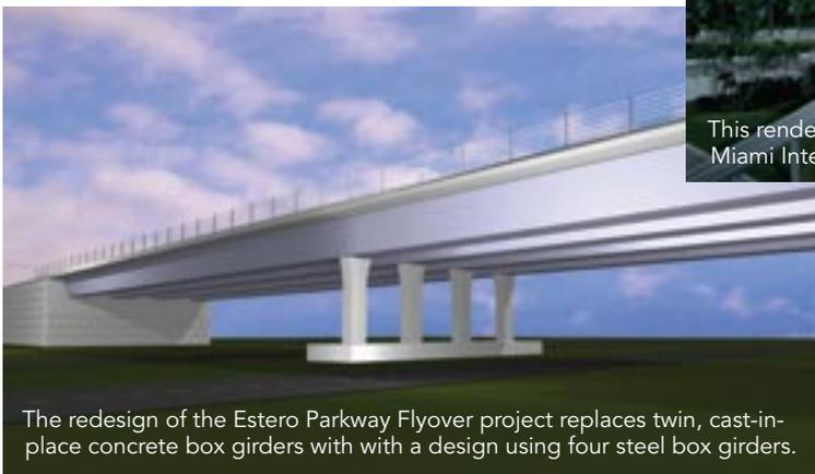
The redesign of the Estero Parkway Flyover project replaces twin, cast-in-place concrete box girders with with a design using four steel box girders.
