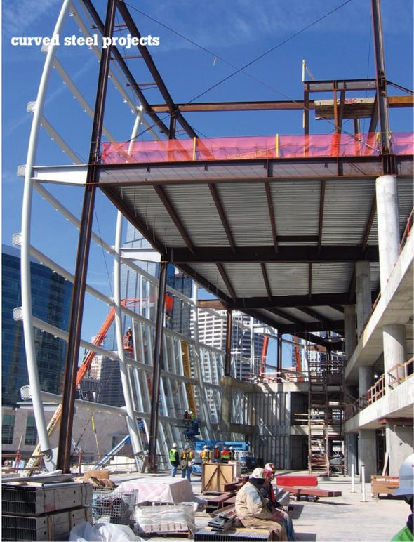
Construction tolerances for the curved steel frame were reduced from those in the AISC Code of Standard Practice to facilitate connection of the cladding system.
