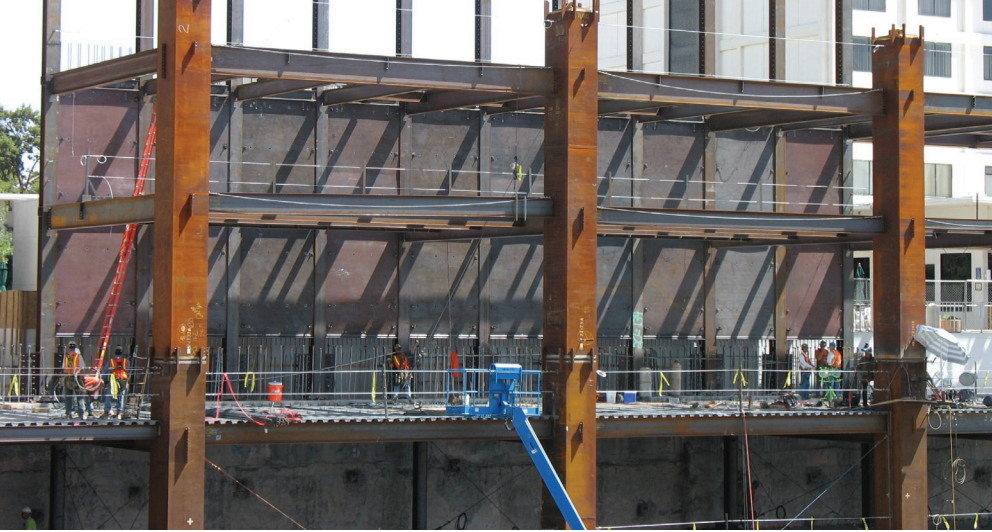
Steel shear walls are used for the lateral system of the Cosmopolitan's podium.
