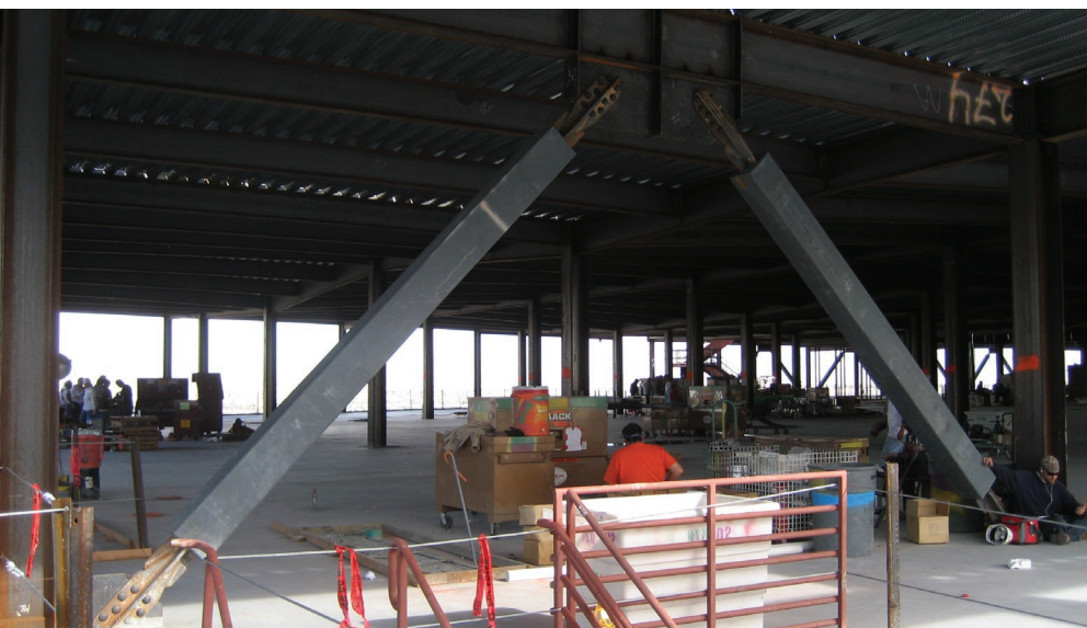
World Market Center Building Three is the first in Las Vegas to use BRBFs.
