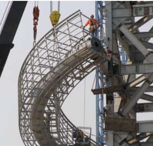
Steel being erected for the theater tower.
