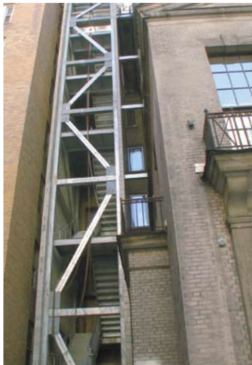
A new egress stair tower at the rear of the building supports two wooden water tanks.
