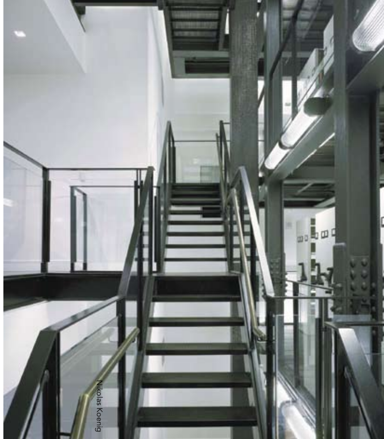
Steel framing is exposed prominently in this structural renovation project.
