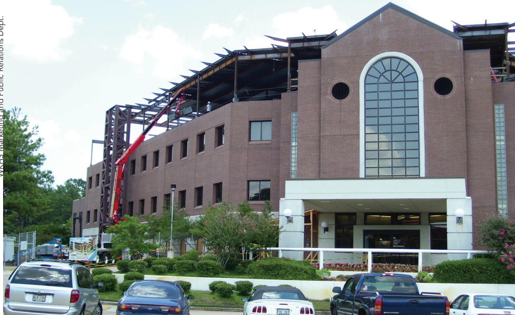
The NICU addition to Shreveport, La.'s South Park Hospital is a braced seismic tower composed of HSS16x8x \frac{3}{8} for all vertical members and HSS8x8x \frac{3}{8} for all bracing and horizontal members.
