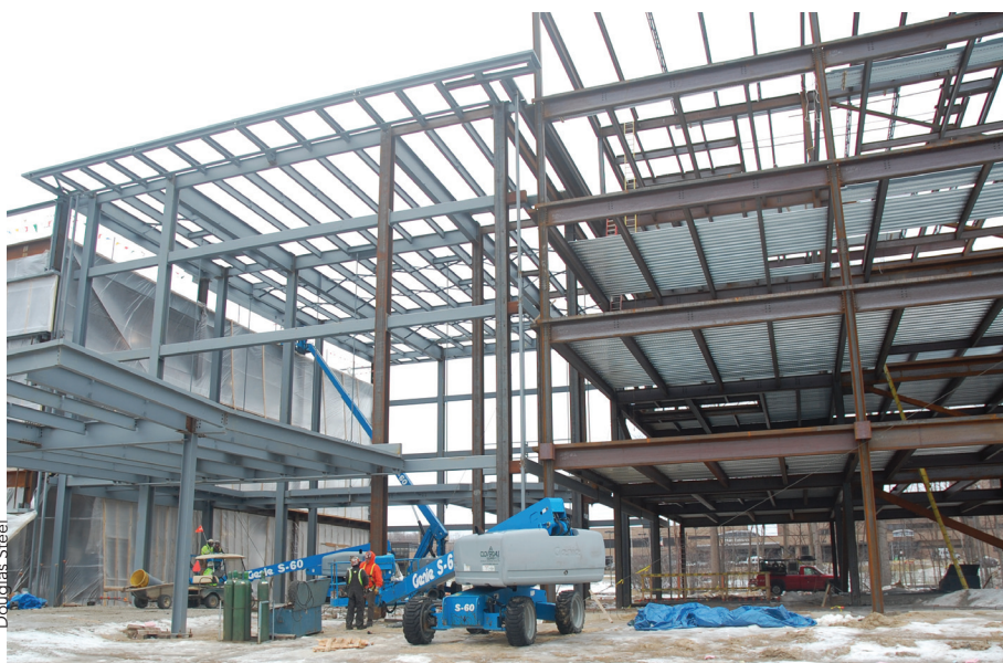
Beaumont Hospital's framing system is constructed with composite steel beams, and lateral resistance is provided by moment frames in the longitudinal direction and braces in the transverse direction.
