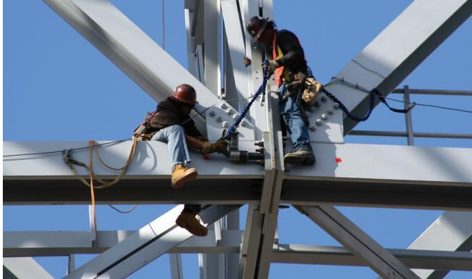
Ironworkers tighten bolts in one of the slip-critical end plate splice connections that link the 56-ft long segments of the arch truss chords.
