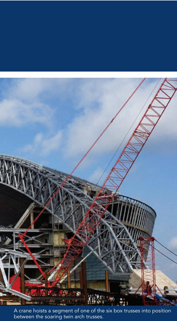
A crane hoists a segment of one of the six box trusses into position between the soaring twin arch trusses.
