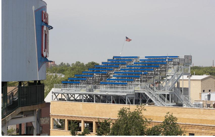
The bleacher system's beams and columns sit on the building's existing load-bearing masonry walls and a new concrete roof (left). From across the street from Wrigley Field, 200 fans can get a clear view of the action (right).
