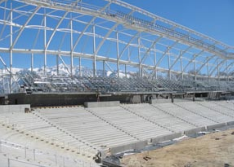
Roof framing before canopy installation.
