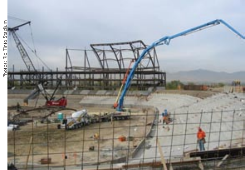
Erection of the canopy framing.
