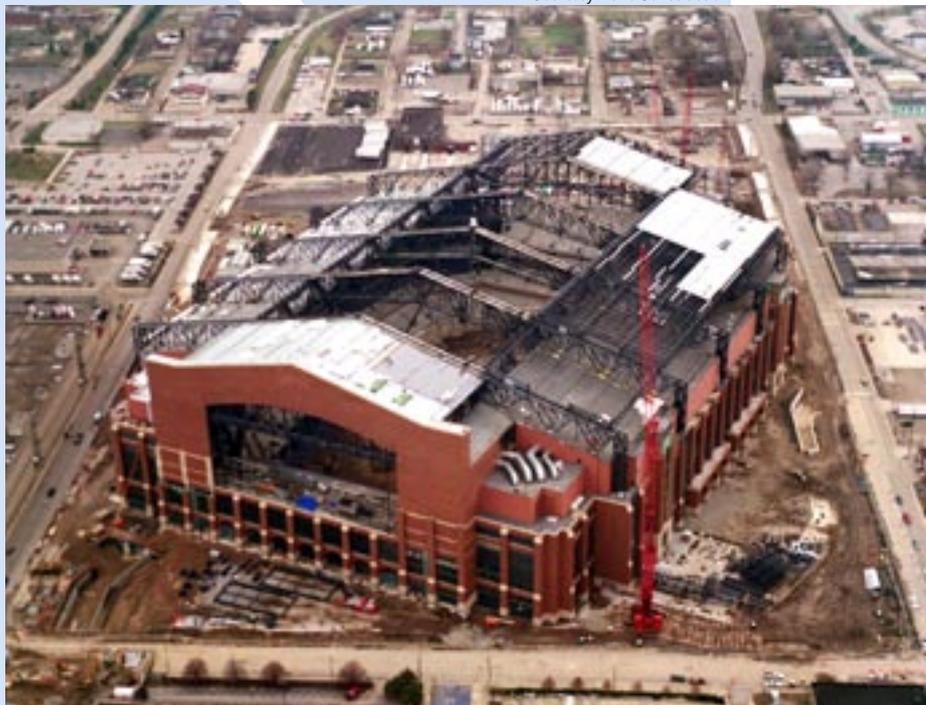
To create the pitched roof that evokes a traditional Indiana field house, the panels were oriented to slide perpendicular to the field sidelines.
