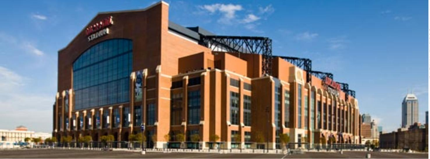
Five transverse trusses span 300 ft to create a distinctive exposed structural form. This first-of-its-kind structural layout eliminated the need for the retractable roof to overhang the edges of the stadium. At 752 ft long, the superframes comprise the longest roof span in the country.
