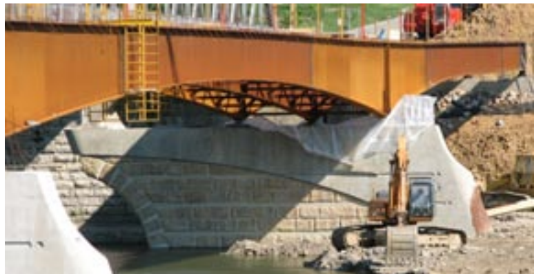
The welded plate girders range in depth from 6 ft at the center of the spans to close to 12 ft at the piers.
