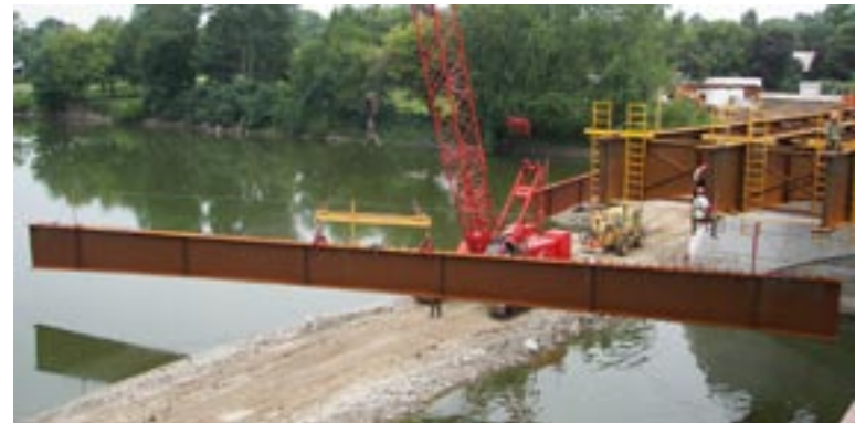
More than 800 tons of structural steel was used in the construction of the bridge.
