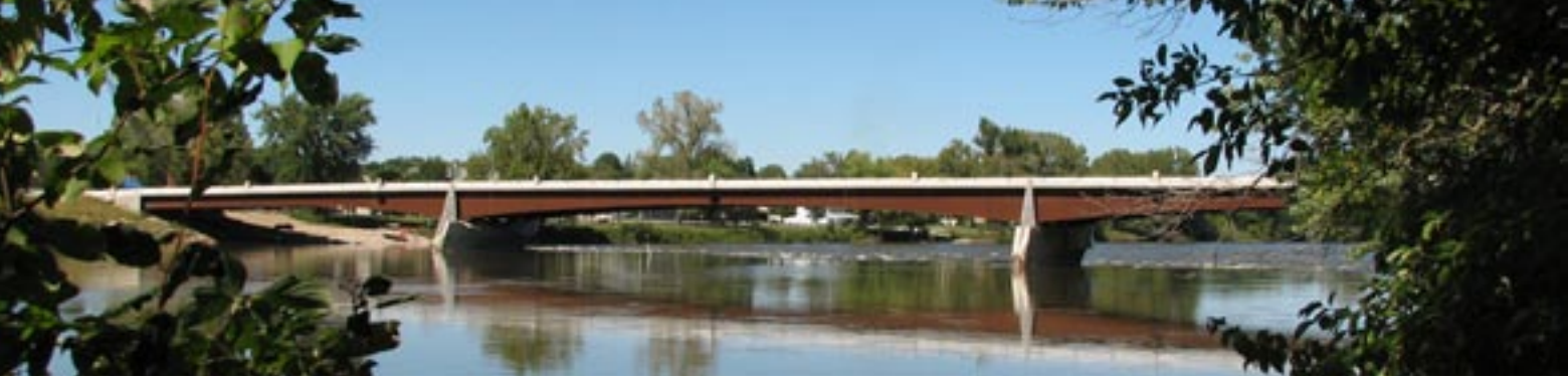
The bridge includes a 32-ft-wide roadway, a 5-ft-wide sidewalk, and a 10-ft-wide bicycle path.
