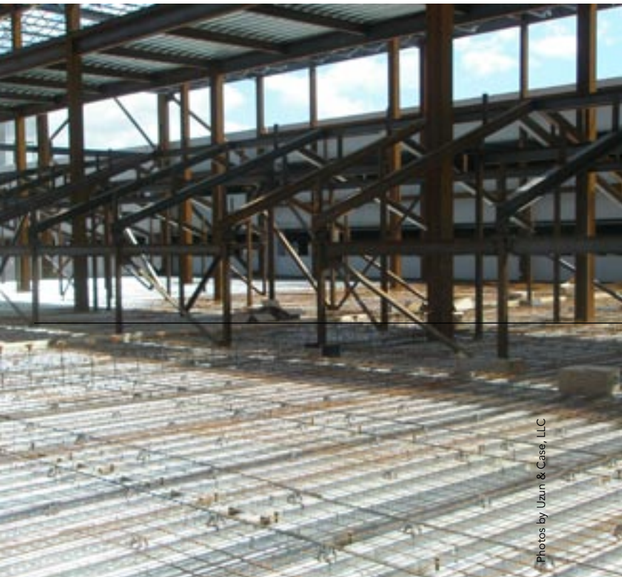
Each theater's stadium seating (seen left and above) had to be structured independently such that sounds (particularly low-frequency) were not transmitted from theater to theater.
