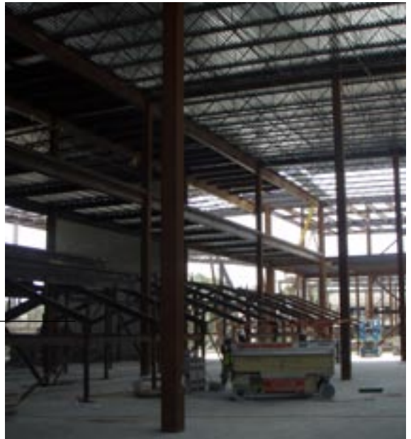
Each theater's stadium seating (seen left and above) had to be structured independently such that sounds (particularly low-frequency) were not transmitted from theater to theater.
