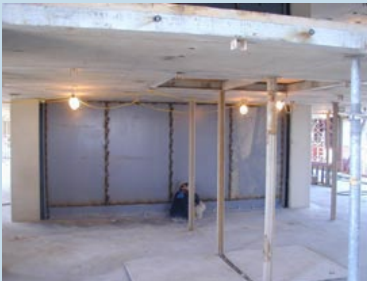
A SPSW in the library's stack tower.
