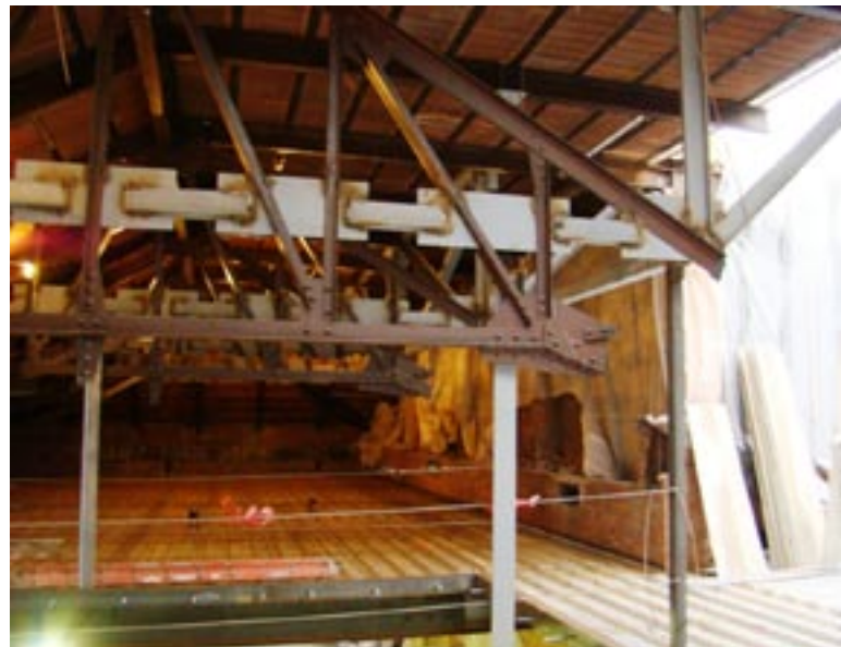
Modifications to the existing trusses in the library's attic.
