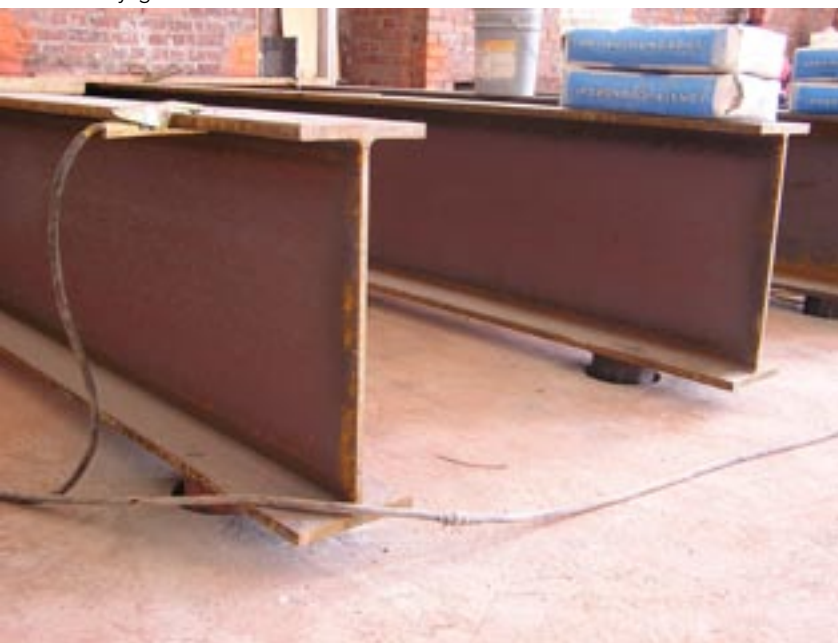
Needle beams for temporary support of the reading room walls.
