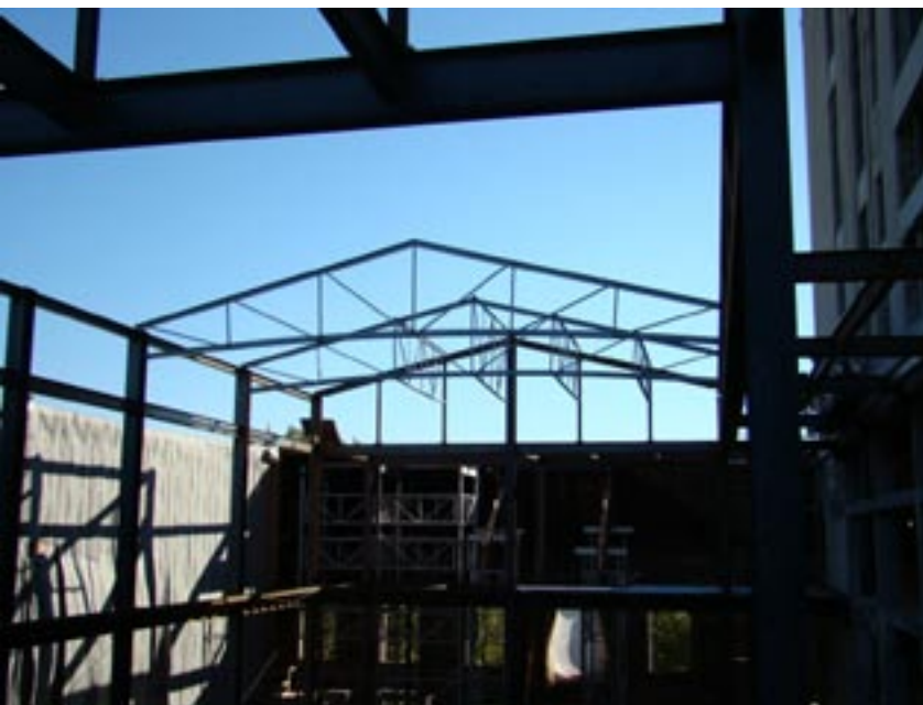
Skylight trusses at the east atrium.
