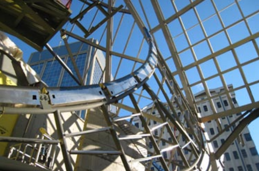
Wide-flange members as large as W14x370, hollow structural sections up to HSS16x16x0.500, and custom box shapes (18 in. by 18 in.) comprised of 1.5-in. plates create the borealis elements.
