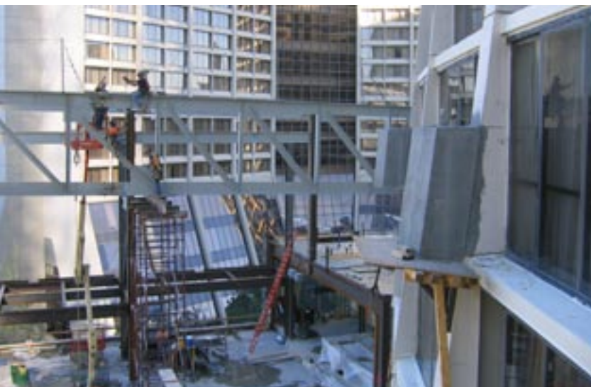
Roof trusses for the Atrium Ballroom.
