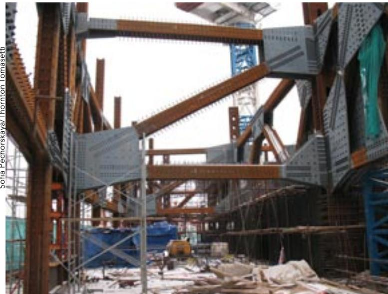
The west section of the 33rd-floor outrigger trusses, linking the belt truss on the left to the central core on the right.
