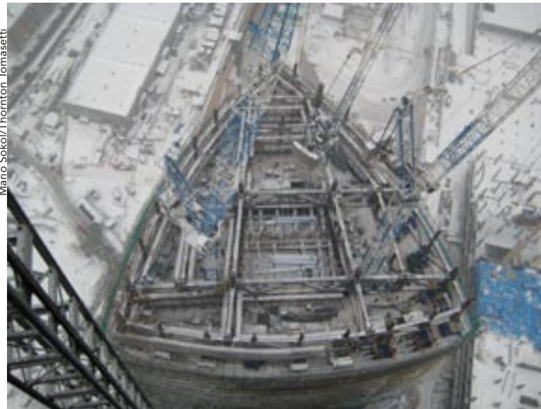
Looking down on Tower A's 33rd-floor outrigger and belt trusses during the final phases of steel erection.
