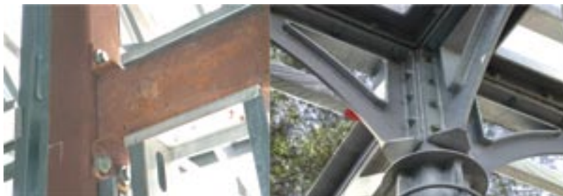
Figure 4: Picture of Hollo Bolt connection details.
