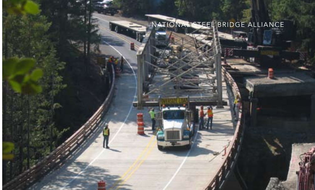
Above: To minimize disruption to its lead-based paint, the 100-ft truss from the old bridge was removed in one piece.
