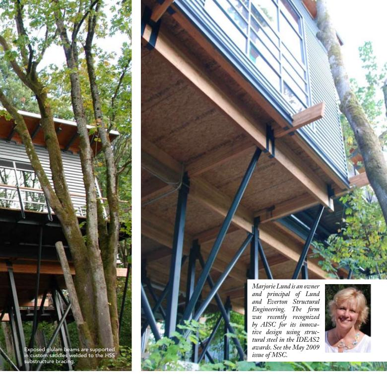
be light on the land through the use of a variety of low impact techniques. Steel piling and a steel substructure support the buildings, thus minimizing damage to tree roots and permitting unobstructed drainage. The use of exposed steel frames below the floors of the buildings and boardwalks minimize the disruption to the site and provides a unique lofty visual appearance.
