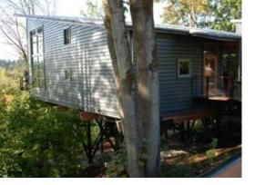
three-dimensional steel and wood system was optimized by the use of RISA-3D software for gravity, wind and seismic forces. The structures are designed for Structural Occupancy Category II in Seismic Design Category D.
