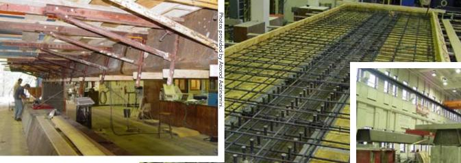
**Fig. 2** Conventional forming materials and methods can be used to form the concrete deck on the folded plate girder.
